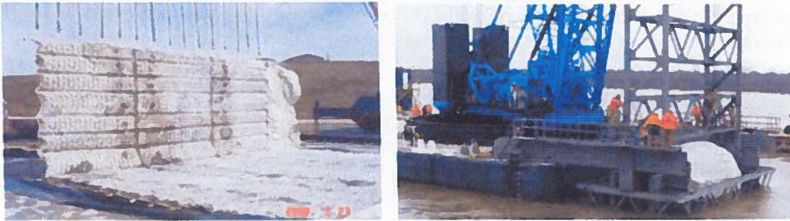
Installation of Pre-Fabricated Seabed Protection System
